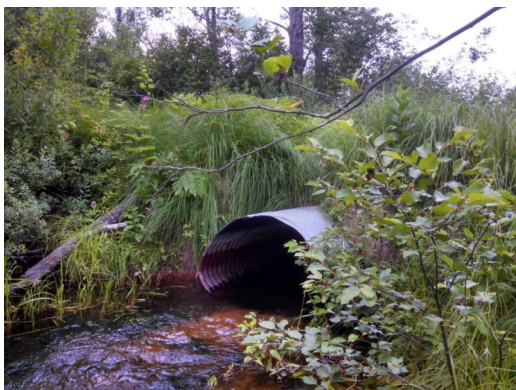
Undersized culvert on Pickerel Lake Road
